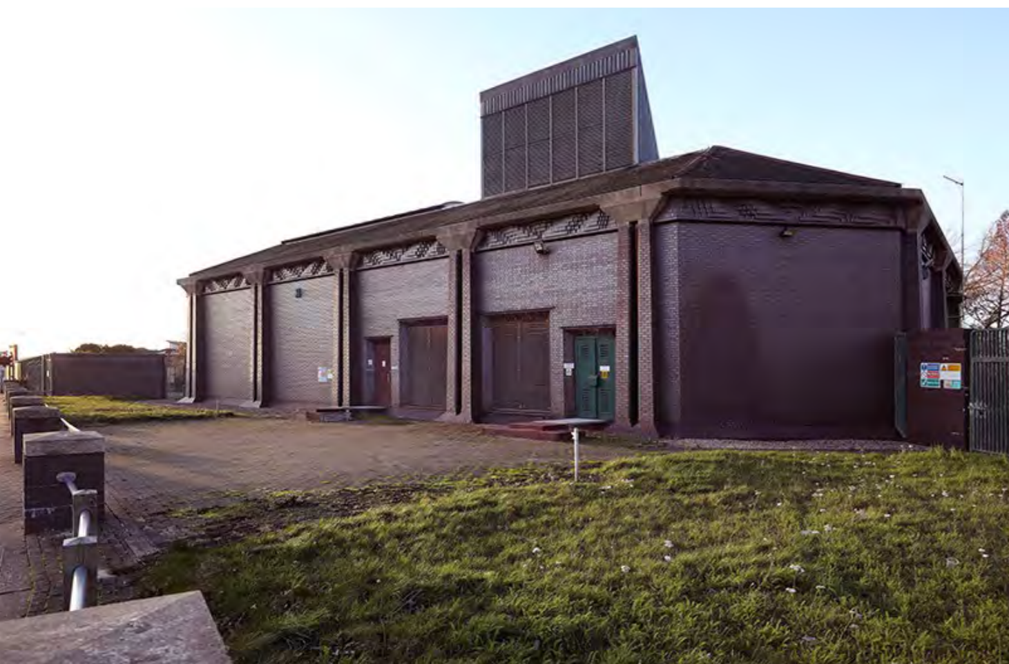
The pumping station at Kings Road, Cleethorpes (see page 24)
